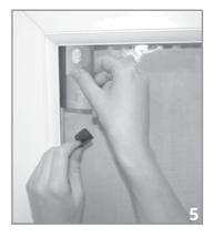
(5) Line up the window fixing bracket at the base of the card (or top of the card depending upon which corner of the window you are working) and fit the bracket by pushing it between the glass and the rubber seal on the window.
