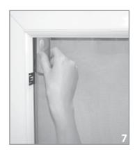
Sit any intermediate brackets accordingly. Clean excess lubricant from window surface prior to fixing frame to brackets.
